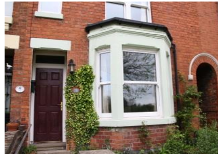
Good brickwork and windows
