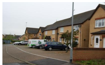
Good parking arrangement
